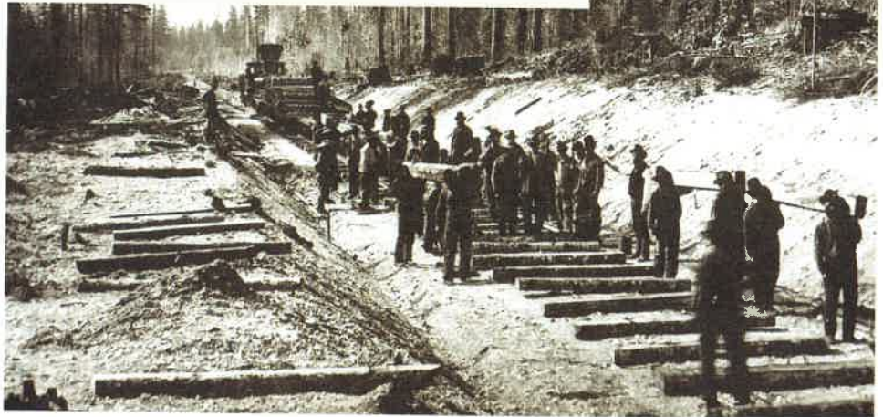
Figure 5-19 Laying the railway ties was exhausting work.
